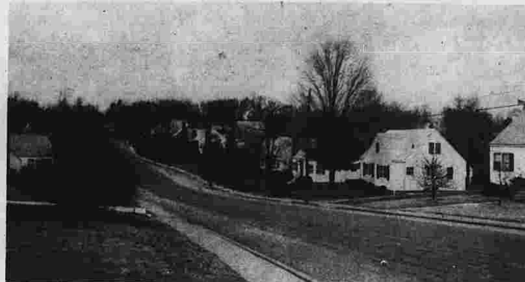
Grant Road shows an example of post-World War II housing development. (Herald photo by Pinto)
